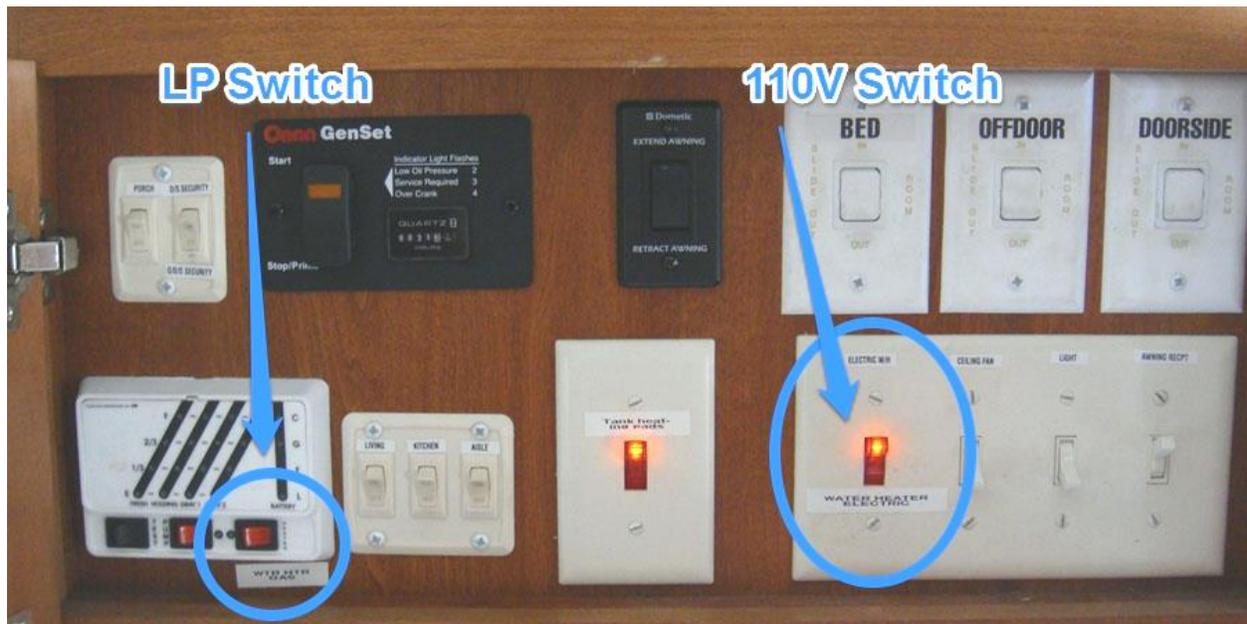
This picture is from a Landmark. Other brands will vary in what's included and where the switches are placed. In most trailers, the 110V switch is similar to a standard light switch, but lights up when turned on. The LP operation is controlled by a smaller rocker type of switch.
