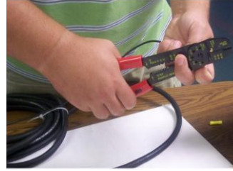
Figure 4.16 Strip ¼” insulation
