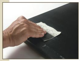
Fill the gouge with the 105 adhesive caulk.
