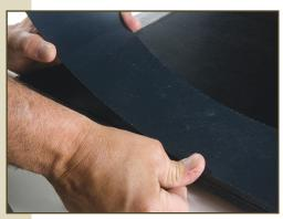
Roll the strip to flatten the adhesive beads and make a good bond with the floor.
