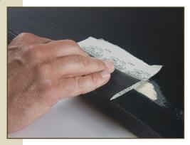
Apply the 105 adhesive caulk to the back of the strip.
