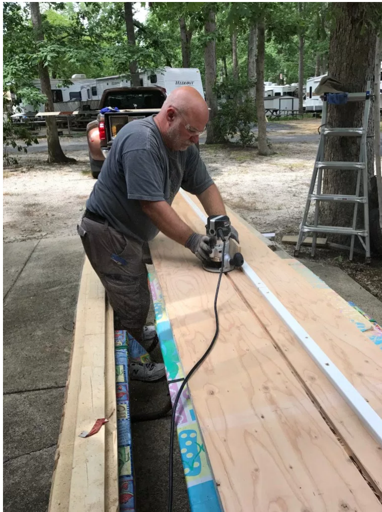
Using router to create 3" lap joint
