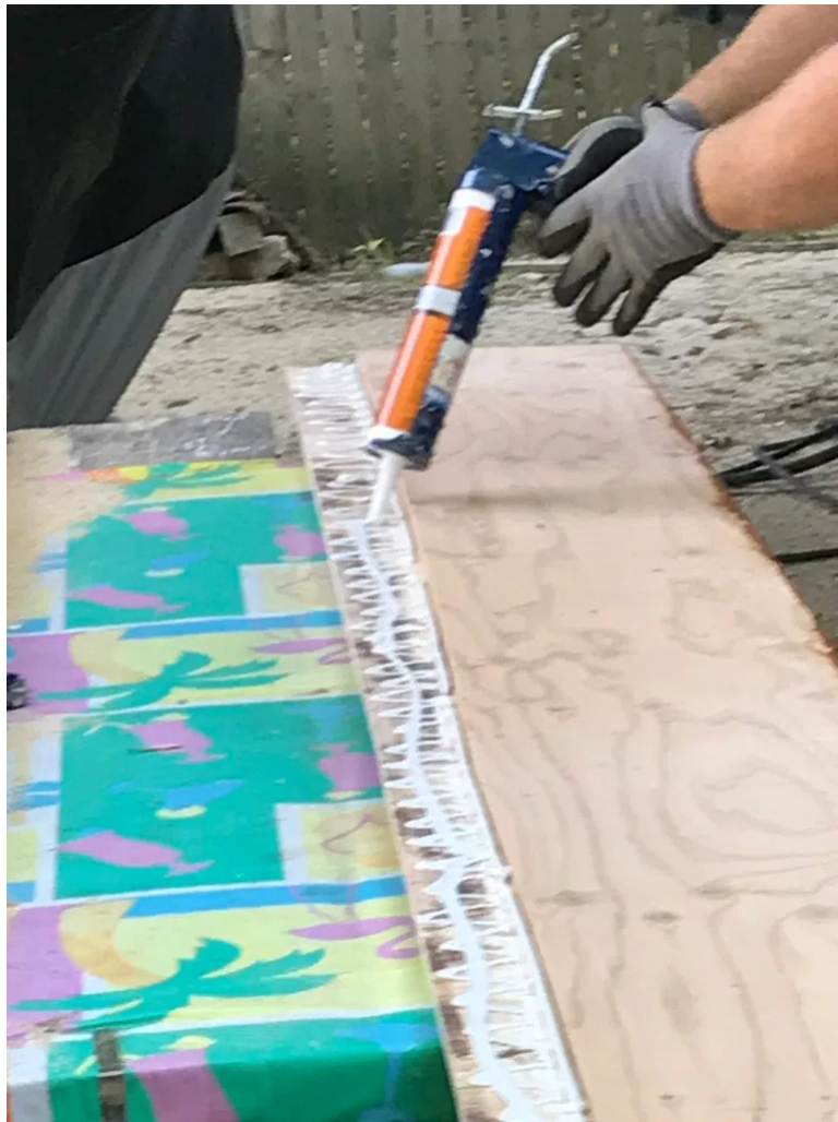
Applying wood glue (Gorilla construction adhesive)
