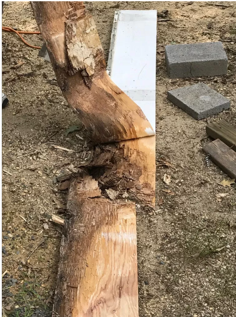
Outside plastic covering pulled away showing totally rotted wood
