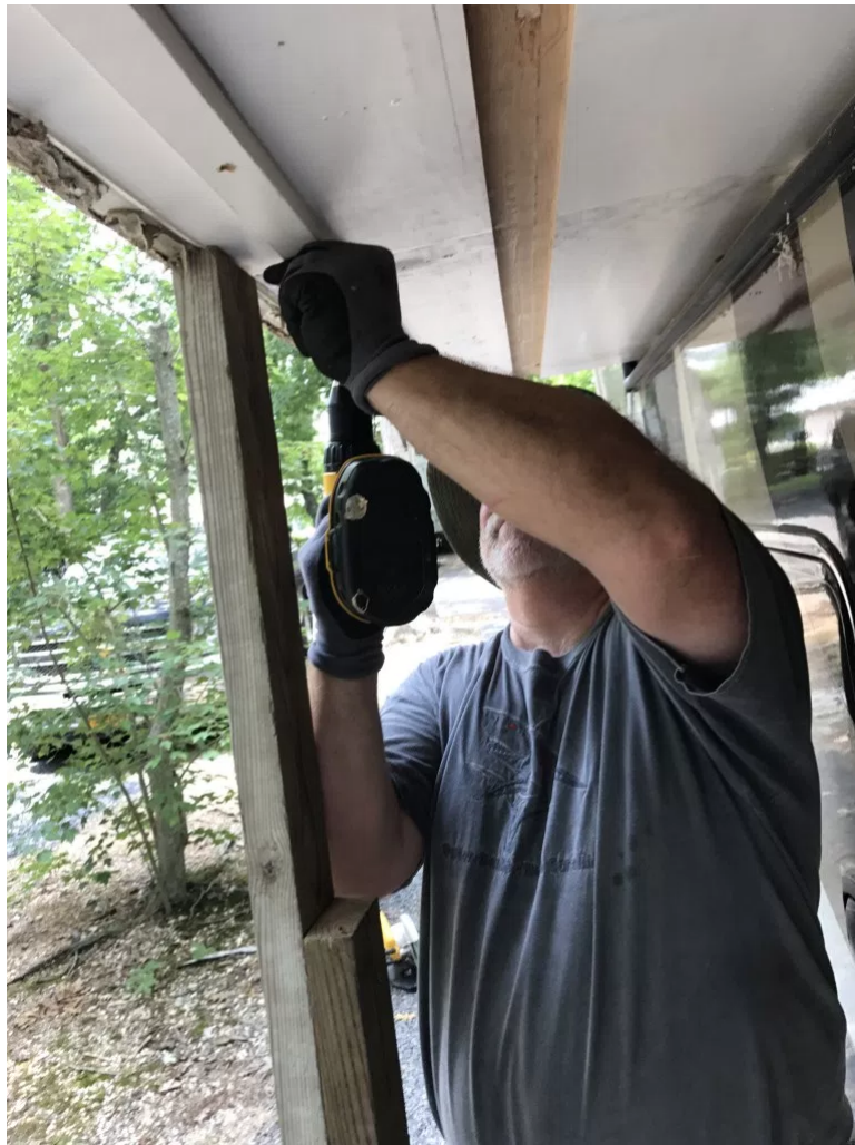
Attaching the guide to cut away damaged floor
