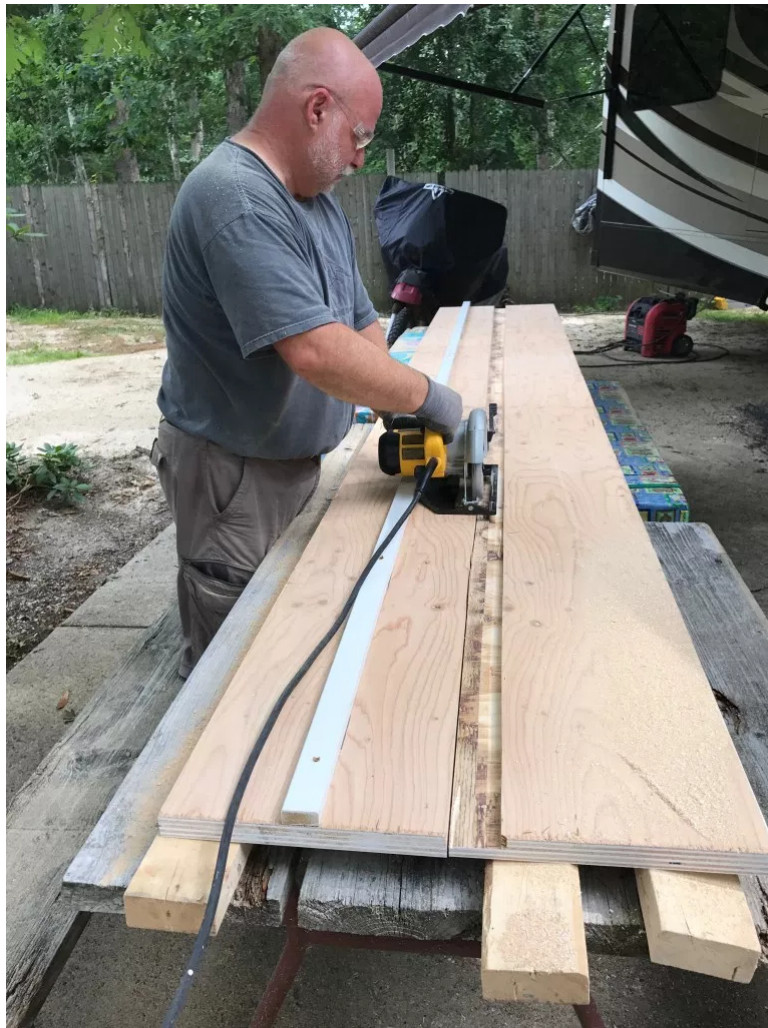
Cutting the floor to size
