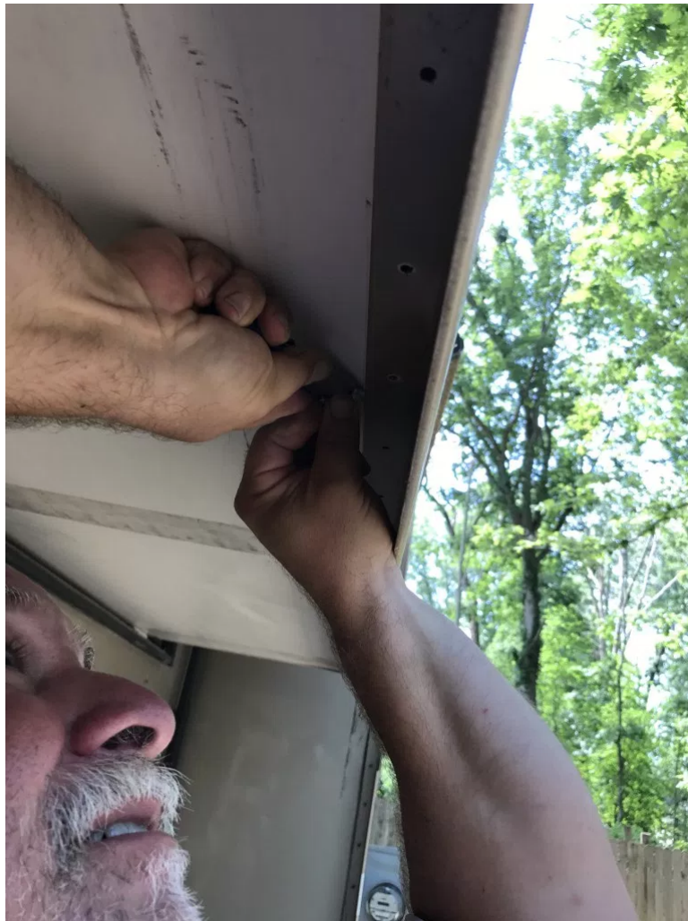
Separating the floor from the trim piece
