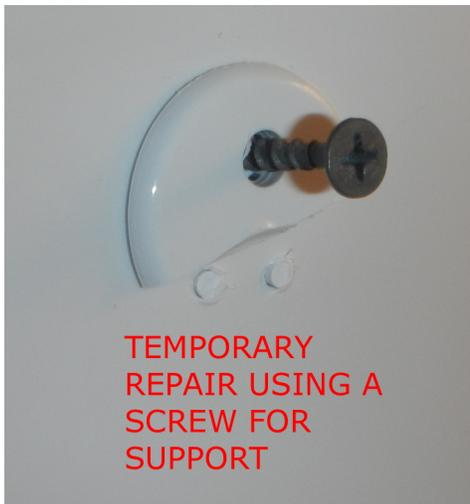
TEMPORARY REPAIR USING A SCREW FOR SUPPORT
