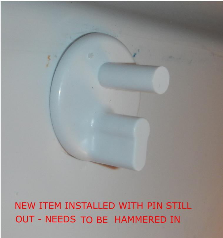
NEW ITEM INSTALLED WITH PIN STILL OUT - NEEDS TO BE HAMMERED IN
