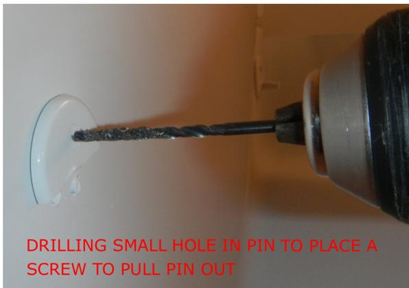
DRILLING SMALL HOLE IN PIN TO PLACE A SCREW TO PULL PIN OUT
