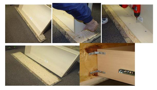
To **reattach the drawer**, center the new drawer in between the marks you made on the kickboard, or between the L brackets you left. Make sure the bottom edge of the drawer is against the  $\frac{1}{2}$ " wide wood stop on the backside of the kickboard, and that the L brackets from the backside of the kickboard are against the sides of the drawer.
